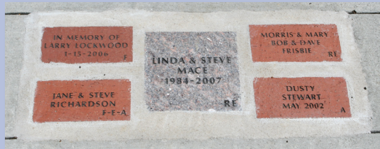
A section of pavers installed on the Ottumwa Campus
